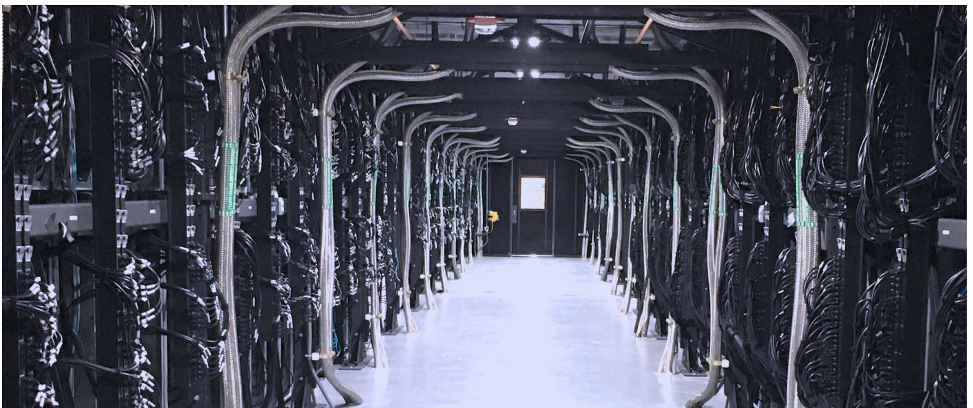
A close-coupled, evaporative cooled, Gen 3B data center hot aisle with 60U racks with up to 280 disaggregated servers/rack and up to 43 kW/rack.
